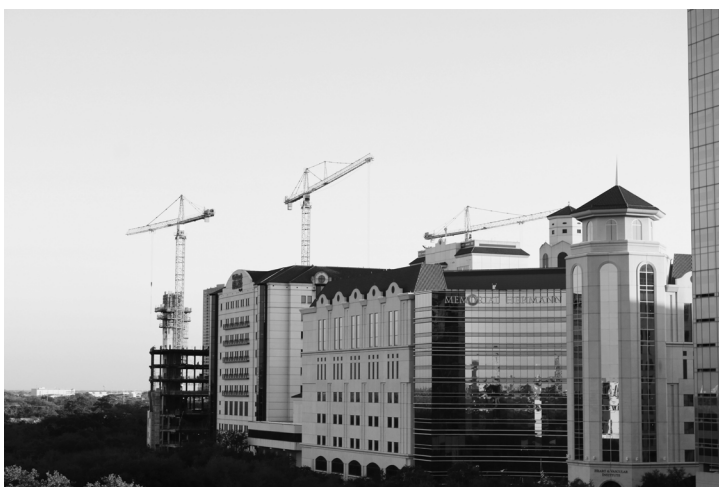
Constructing. Photo by Ginny Jeon.
